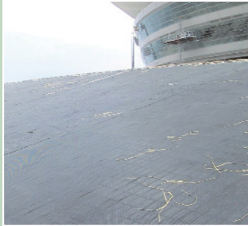
Singapore - Punggol East Public Housing Project, multistorey car park and roof garden
